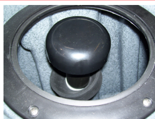
Float Shutoff Assembly
